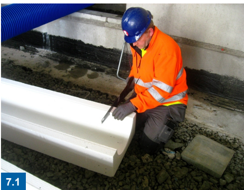
Adjustment with hand saw
