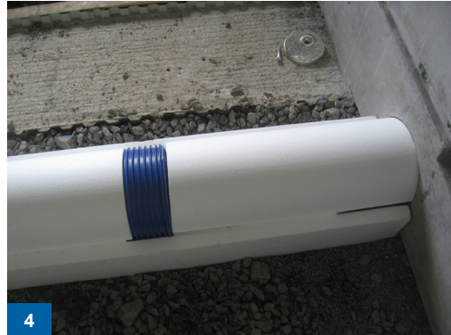
Inset is placed on top of the ducts
