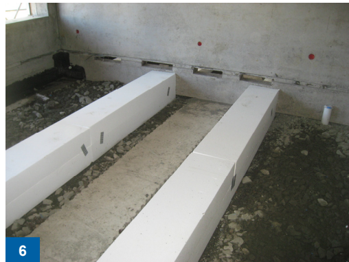
The top section is fixed with toothed-plate connectors
