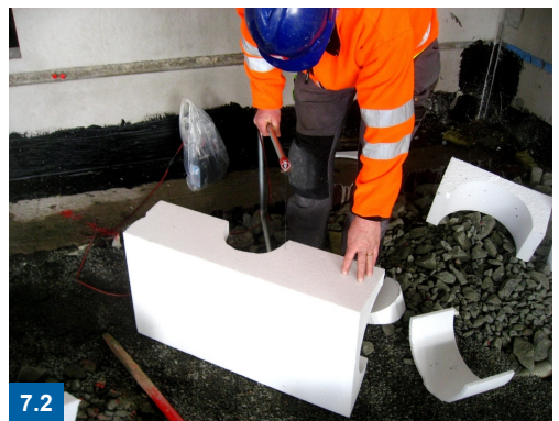
Adjustment with hot wire
